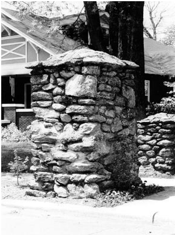
The rock columns have proudly stood at the entrance
