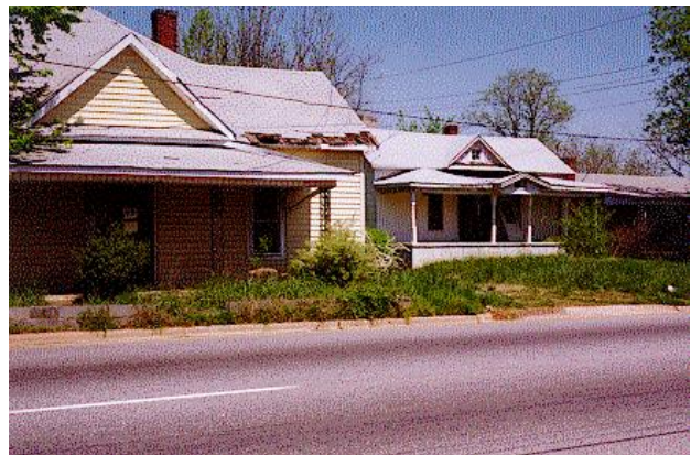
These two dilapidated rental houses on First Avenue SE were condemned in 1995 and have remained vacant since.
