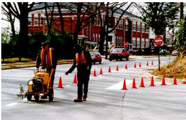
Traffic Division co-workers paint pavement markings at a dangerous intersection in February 1997, three months before the plan was adopted.
