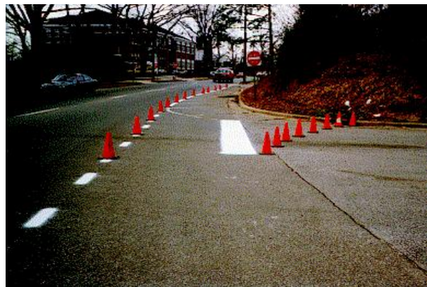
Pavement markings made the intersection safer for motorists crossing Second Avenue SE.
