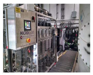
For over a century, water plants have used chlorine gas. It is a very good disinfectant, but safety is a major concern in its use and handling. Many water plants have switched to sodium hypochlorite as a disinfectant. Most plants have concentrated commercial grade delivered by truck, but Hickory was the first in North Carolina to purchase its own sodium hypochlorite generator.
