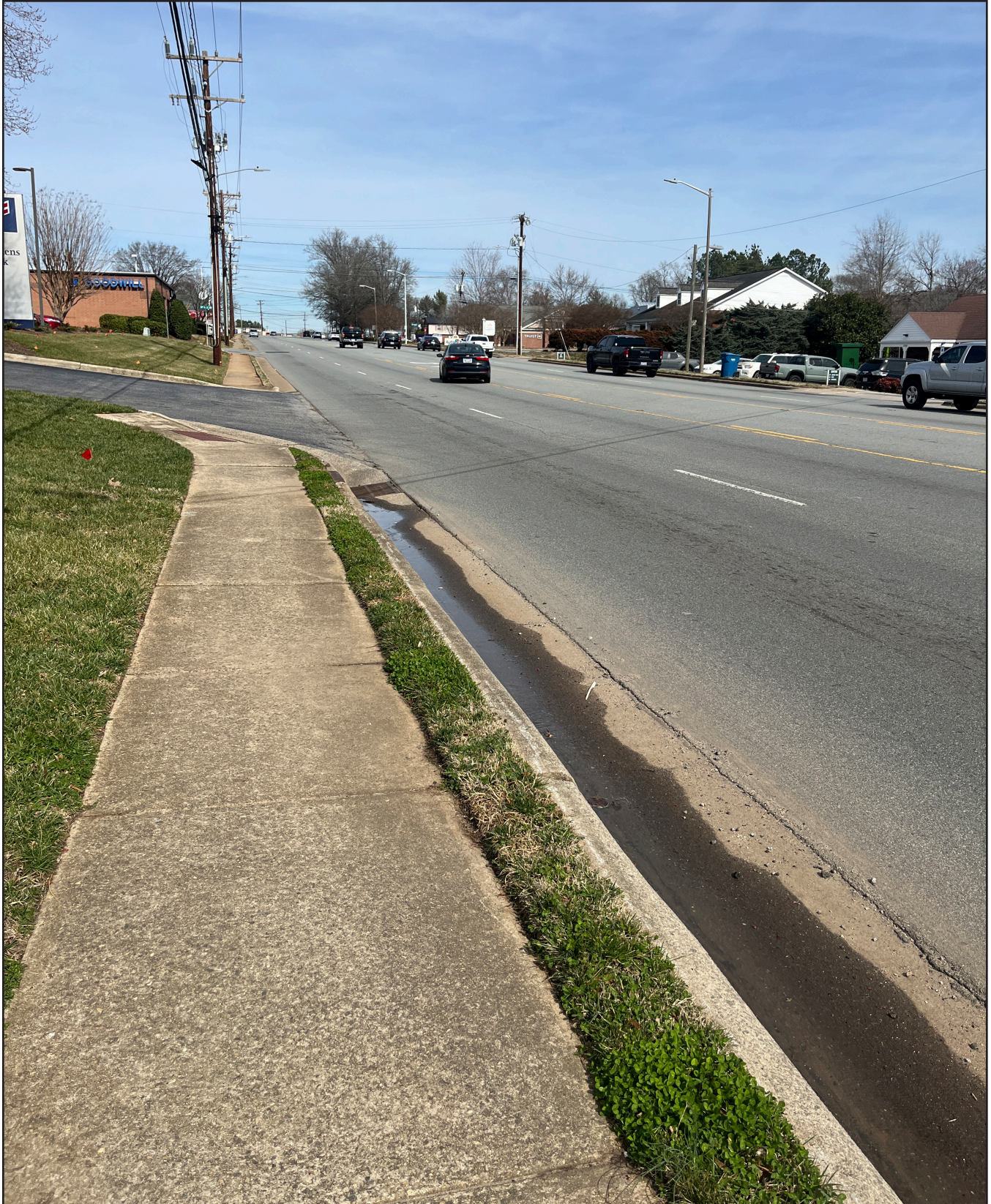
NC-127 and 18th Ave Dr, facing north
