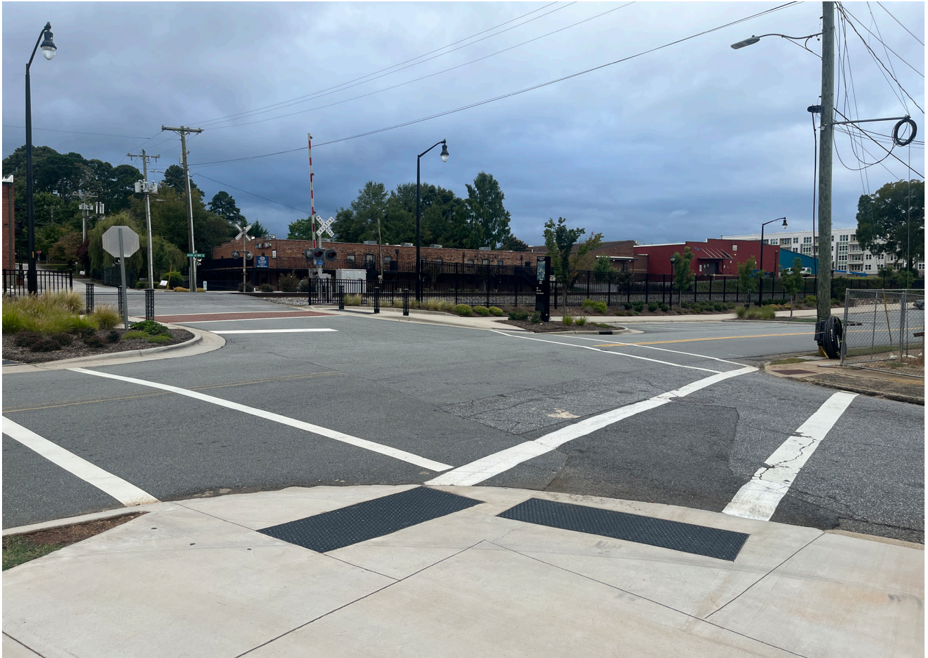
Main Ave NE and 2nd St NE, facing City Walk trail crossing
